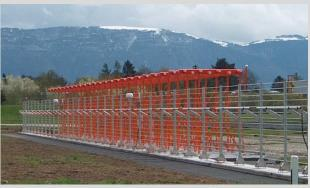
Antenna is Shown with a Park Air Systems LPD Array Used for Clearance Signals
