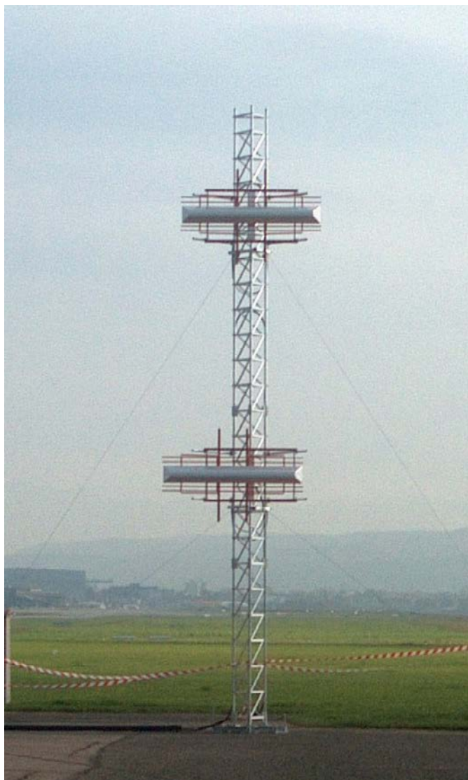
Watts Antenna Company's Model GP5-A1 Image Glide Slope Antenna. Initial testing of Model GP5-A1 and GP7 family of antennas was successfully flight tested in Zurich, Switzerland, for Category III operations in November 2006.
